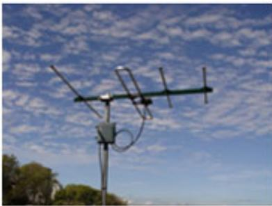
Mast head amplifier too close to the antenna
