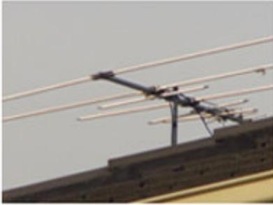
Antenna installed too close to roof
